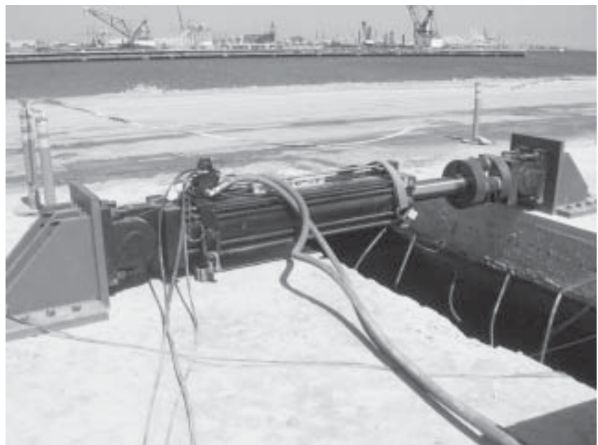
A hydraulic piston bolted to two sections of the pier slowly expands, subjecting the pier to lateral loads that might be experienced during an earthquake. Photos: UC San Diego, Department of Structural Engineering
